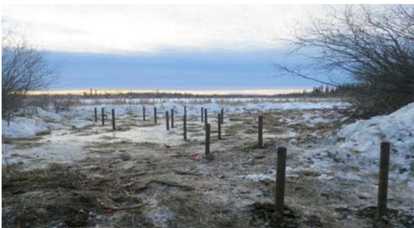
**Screw piles in place before blind construction can start**
